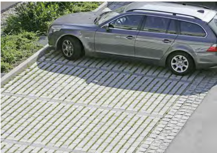
Permeable parking space
