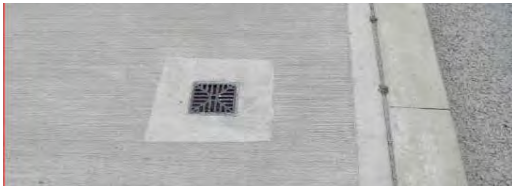
LIGHT GREY CAST INSITU CONCRETE (BRUSHED)
